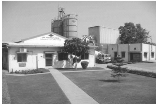
Fig.2 A modern eco friendly RMC plant with advanced manufacturing process and technology for producing quality ready-mixed concretes
