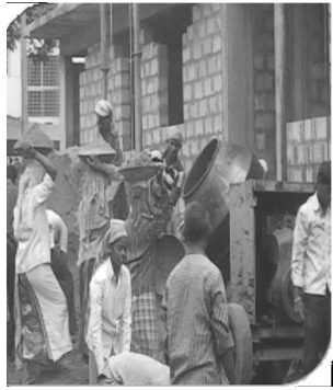
Fig.1 Traditional site mixed concrete under usage in India- the most primitive methods of concreting
